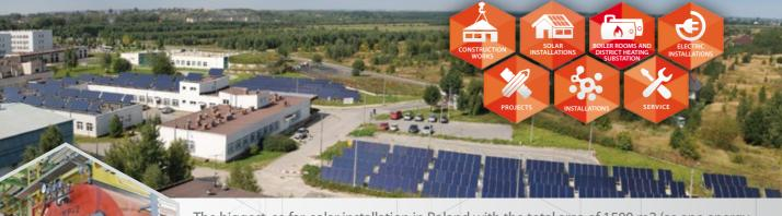
The biggest, so far, solar installation in Poland with the total area of 1500 m2 (as one energy system) and one of the biggest installations of this type in Europe. 598 pcs. of solar collectors were mounted partially on hospital building's roofs and partially on free standing structures.
