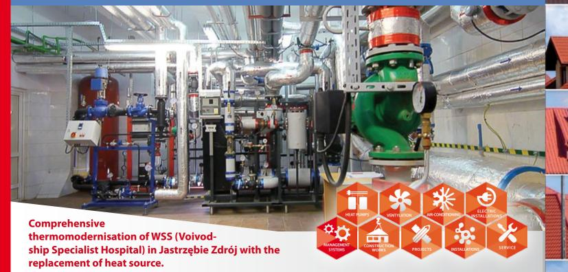
Comprehensive reconstruction of the heating system including i.a. replacing existing heat source with a cascade of three heat pumps of 716 kW with the use of the ground heat source as 102 bores of total length of 18000 linear metre. All works were done on the functional hospital facility.
